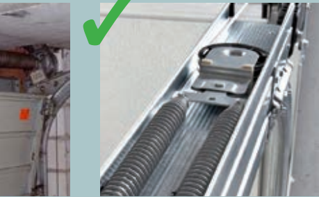
Concealed springs shown from above with the covers removed.
