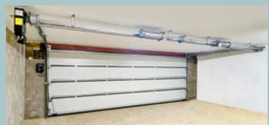
Low headroom rear torsion spring option.
